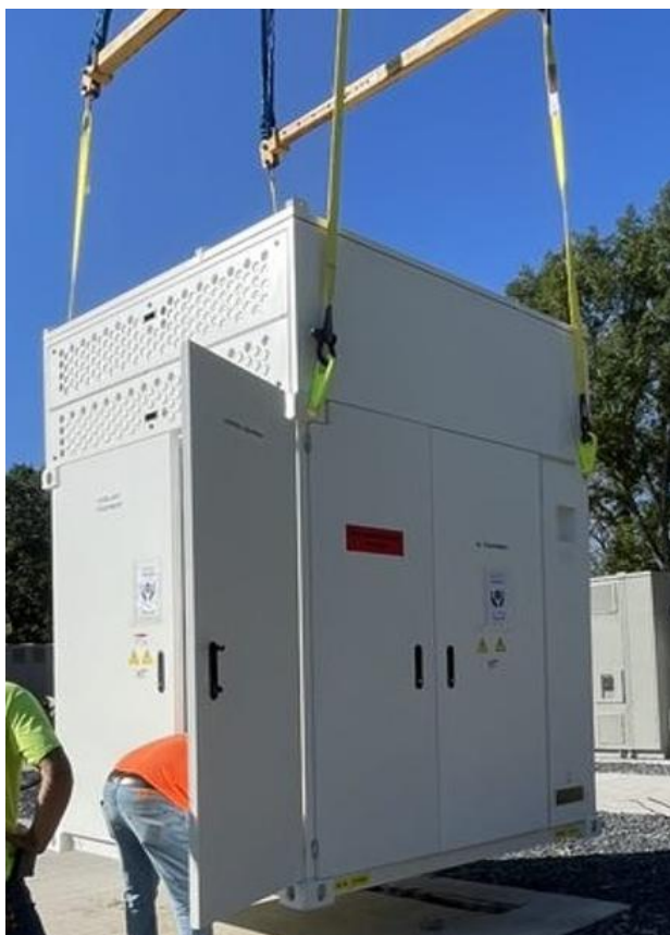
Figure 5.1 An example of a lithium-ion battery unit
